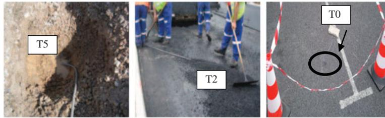
Figure 3. Layout of the temperature sensors.
